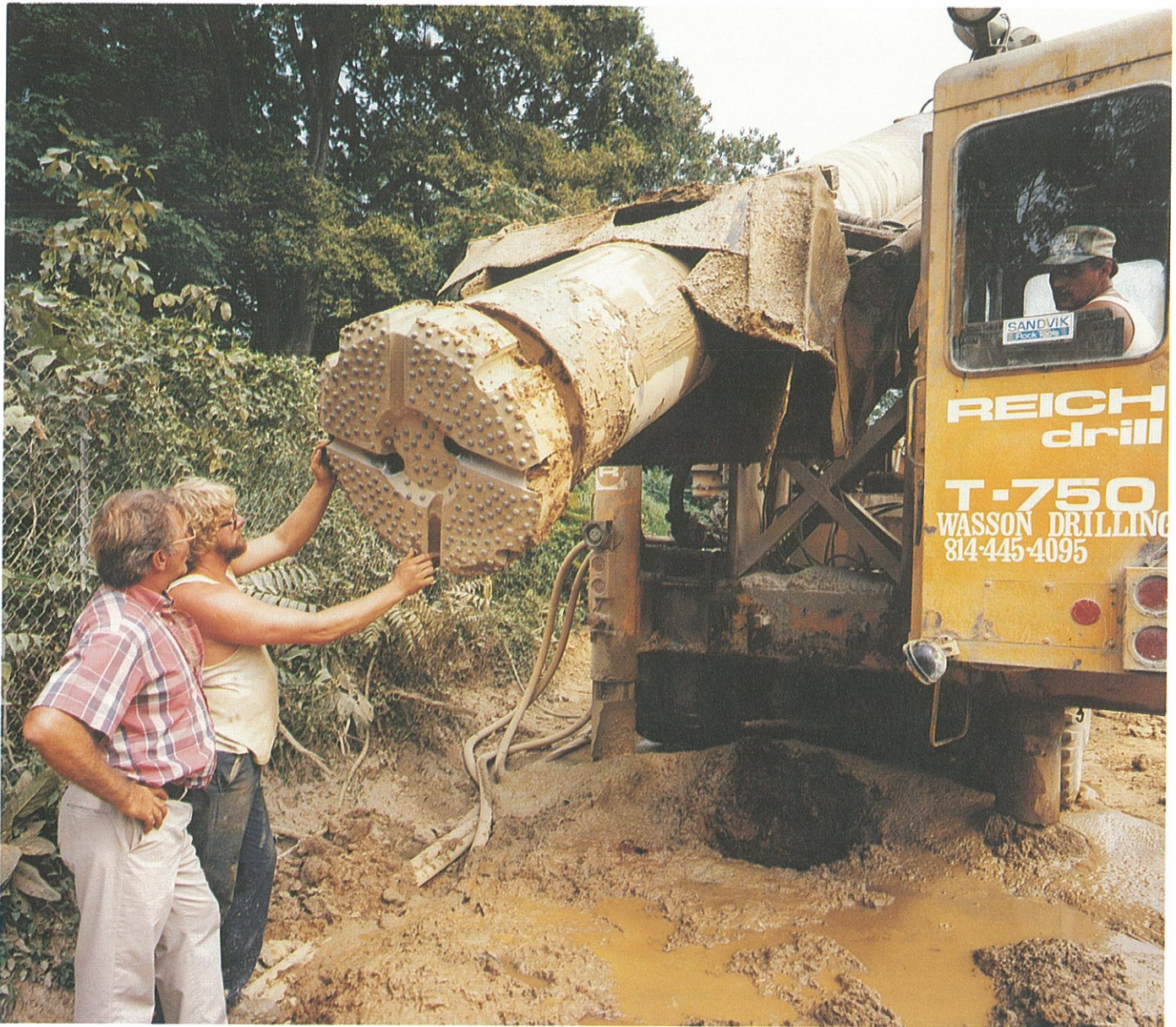
A big Sandvik Mission down-the-hole hammer is being used to drill very-large-diameter holes in the building of a highway outside Baltimore in the U.S.
